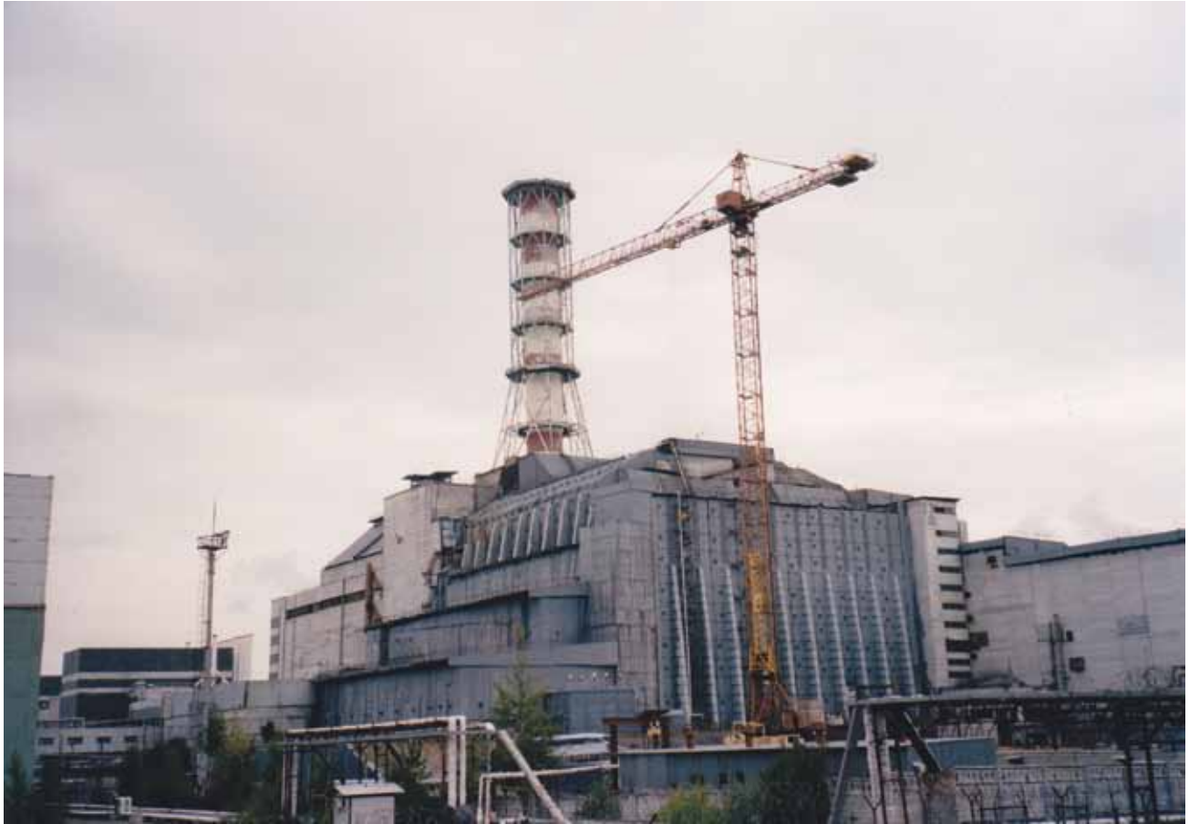
Figure 8-6. The Chernobyl Nuclear Power Plant, where an explosion and fire in the number 4 reactor caused a large release of radioactive materials and a major disaster on April 26, 1986. In the aftermath of the disaster, populations in affected areas have been gripped by a deep sense of fatalism.
